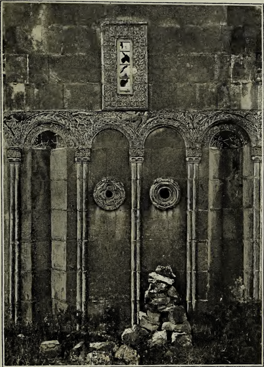
FIG. 77. ANI. NORTH WALL OF THE CHURCH OF ST. GREGORY.
